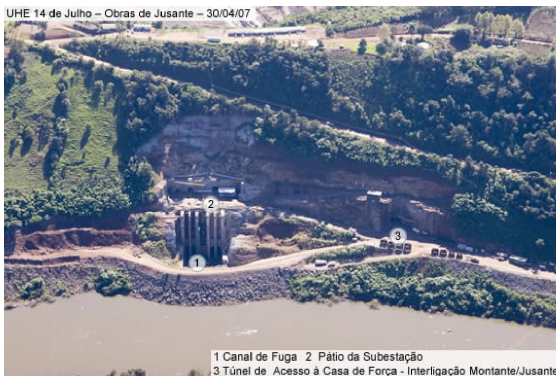
Figure 1 – HPP 14 de Julho ., downstream works. (Source: Ceran)
