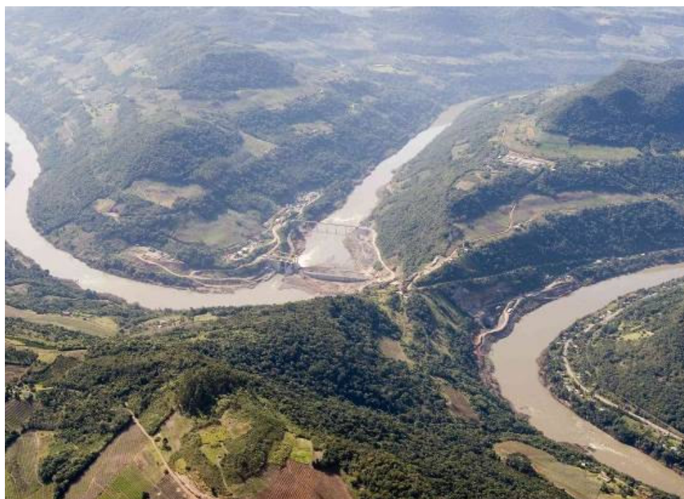
Figure 3.5 – Upstream and Downstream works – Source: CERAN
