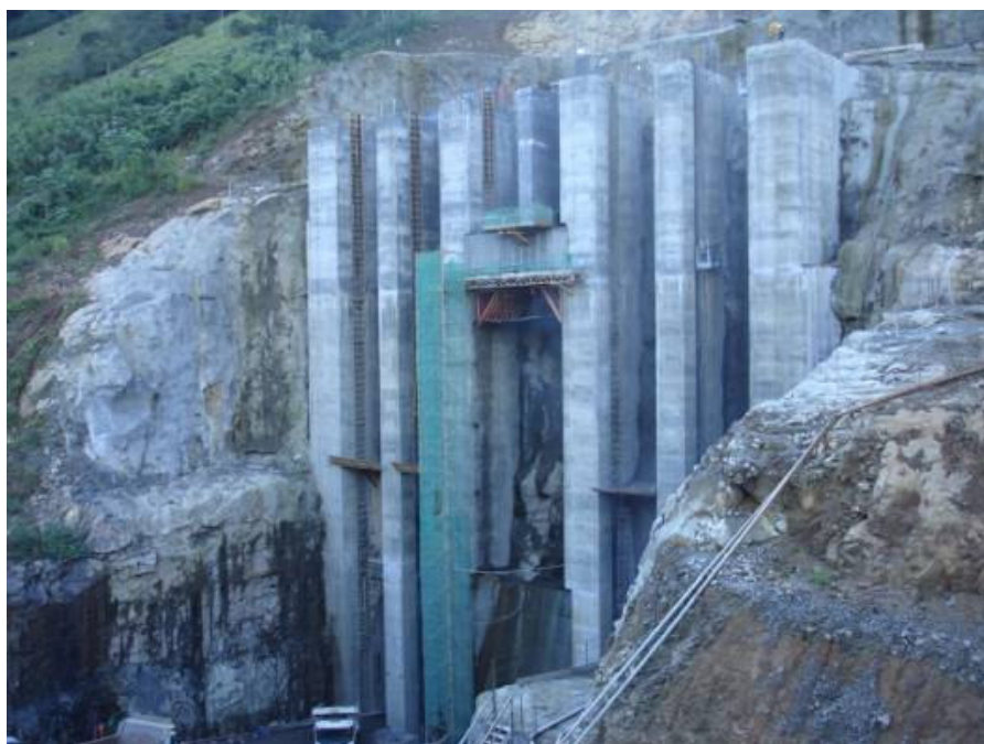
Figure 3.1 – Power House – Suction Structure Construction – Source: CERAN
